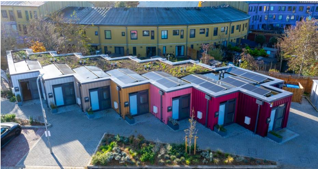
Recent example of a modular rough sleeping accommodation scheme delivered in partnership between the council and a Registered Provider in Aylesbury
