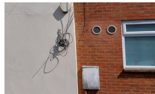
Loose wires and service boxes
