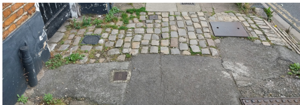
Pavements scars are common across the Conservation Area and detract from its appearance
