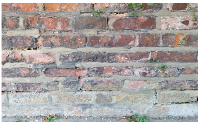
Poorly executed cement mortar repointing
