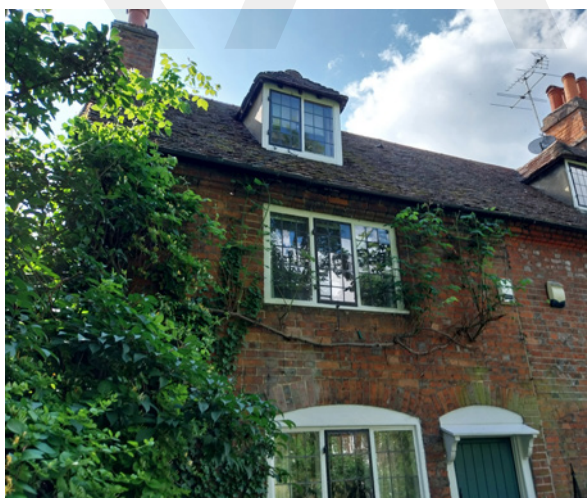
Invasive ivy growth can damage masonry
