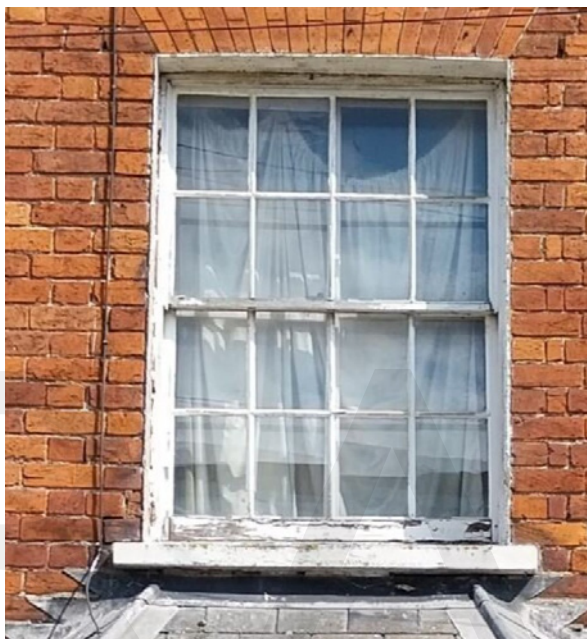
Peeling paintwork on an historic timber window
