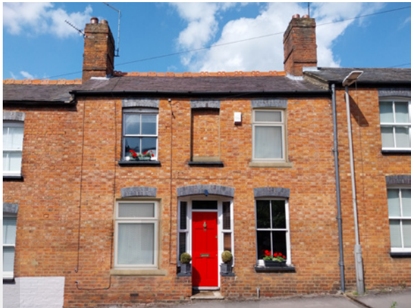
The piecemeal insertion of uPVC windows, which do not follow the traditional glazing pattern and require the widening of openings, skew the proportions of details such as window headers and the symmetry of the building.
