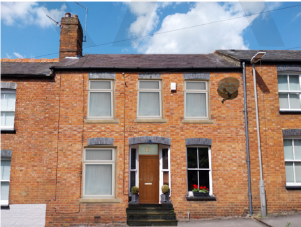
The alteration of original design features in renovation projects, such as the opening of the central blind window and removal of decorative ridge tiles when re-roofing, remove the building's finer architectural features.
