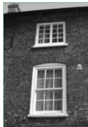
Examples of single-glazed wooden sash and casement windows
