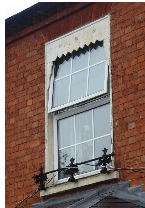
Figure 50 Poor quality, uPVC window in a positive, nineteenth-century building within the Conservation Area
