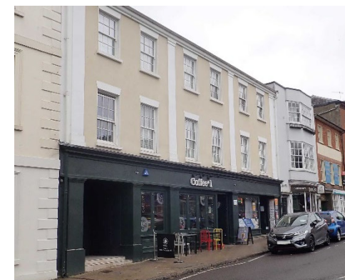
Figure 52 The former site of the NatWest Bank, Market Hill, recently enhanced with a traditional shopfront, timber sash windows and architectural features such as pilasters and a cornice
