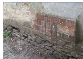
Stone plinth and Rat-Trap bond, brick repairs, Witchert wall, Stockwell
