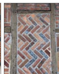
Herringbone infill brick panels at 6, Fort End
