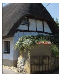
Rendered infill panels
