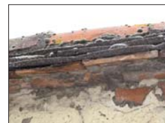
Tiled coping to witchert wall
