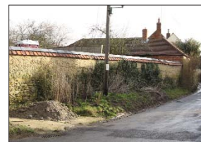
Witchert boundary wall along section of eastern side of lane
