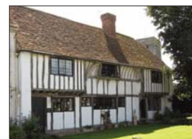
Narrow timber framing at 13, Church End
