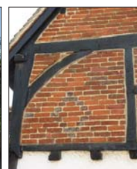
Infill brick panels with diaper work
