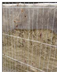
Witchert wall being constructed in berries
