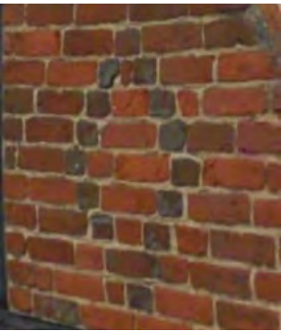
Diaper pattern made from vitrified brick headers at 35 High Street
