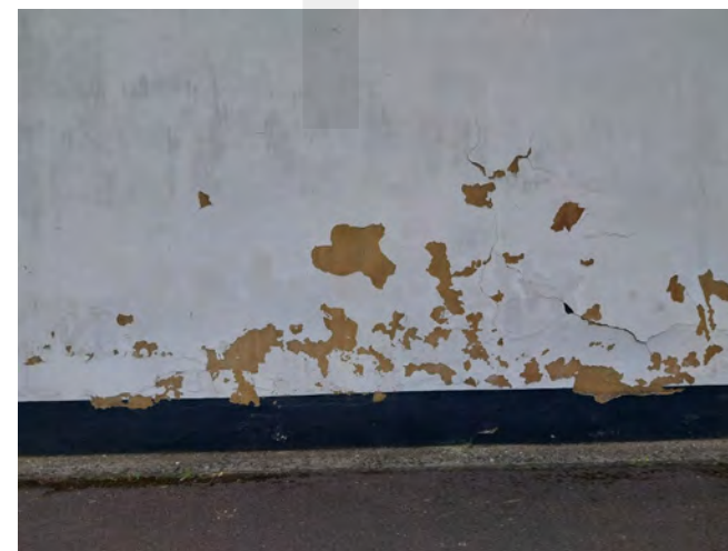
Peeling paint is a common problem on rendered buildings
