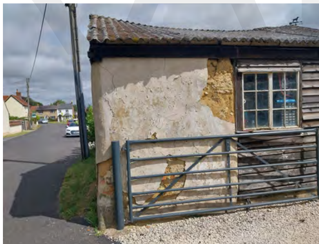
A prominent witchert outbuilding suffering from lack of maintenance, resulting in crumbling render and rotting windows
