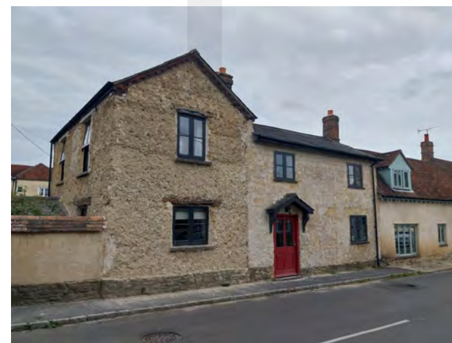
A witchert building with its render removed, showing both traditional mass construction (left) and an extension in witchert blocks (right)
