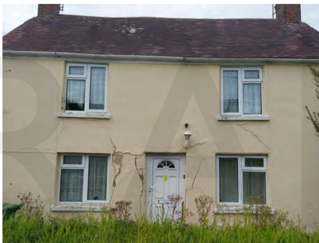
Example of an historic building retrofitted with inappropriate uPVC and impermeable paint, while also showing other signs of major structural failure, likely due to inappropriate interventions
