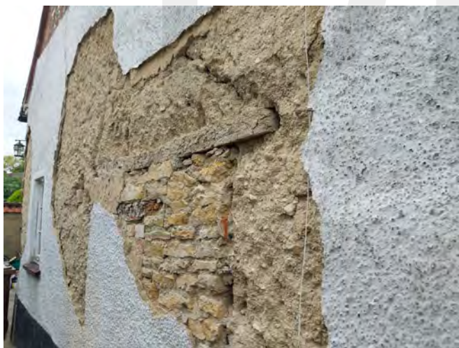
The use of cementitious render over solid wall construction can cause failure and degrading of structures
