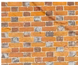
Flemish bond with orange stretchers and vitrified brick headers at Ivy Cottage, Fort End
