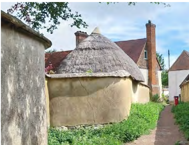
Fruit store built into witchert walls, Duck and Donkey Alley
