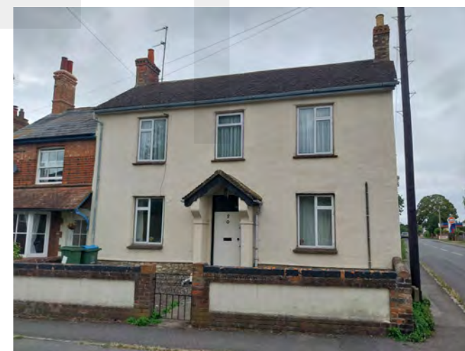
Similar unlisted nineteenth century buildings that have undergone detrimental alteration, including the installation of uPVC windows of inappropriate style and possible cement-based render
