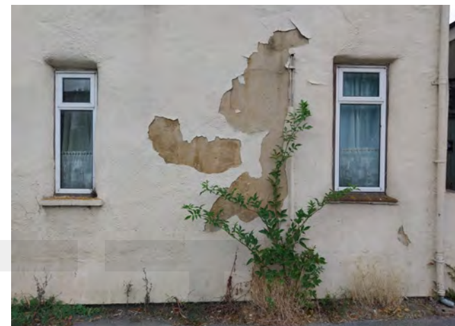
Peeling paint is a common problem on rendered buildings, often due to the poor compatibility of modern impervious paints
