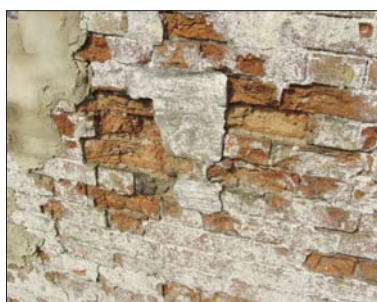
Spalling brickwork
