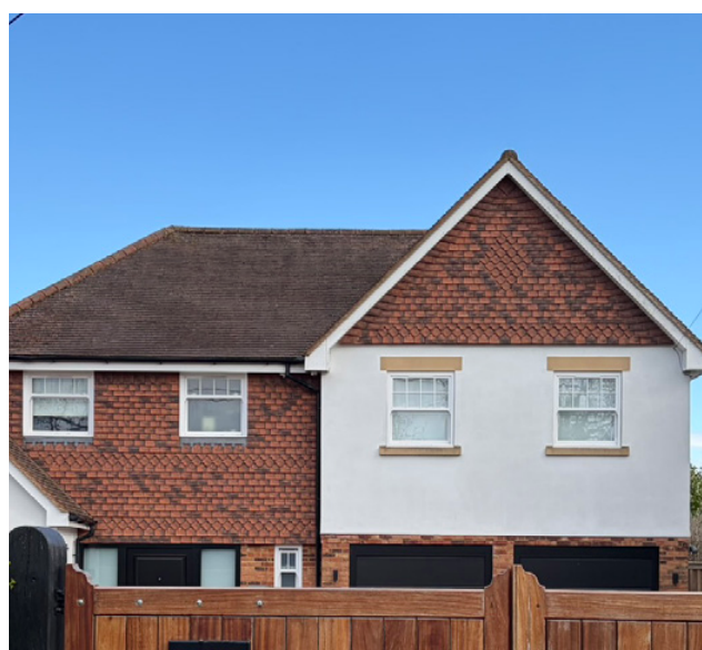
More modern property with a mix of materials, including hanging tiles as an accent on the gable end
