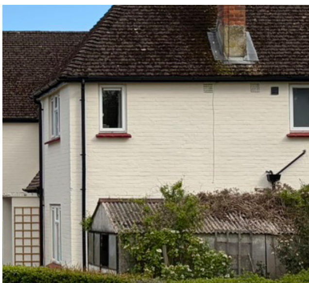
Mid-20th century property where the facing brick has been painted, so the texture shows through
