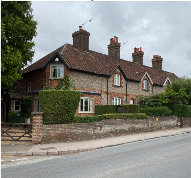
One and a half storey residential properties arranged as a short terrace, in Ashley Green village
