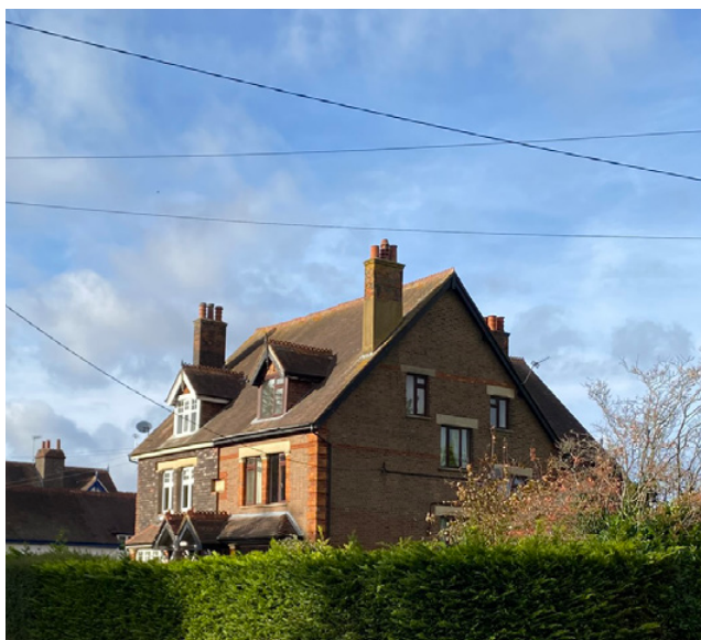
Strong central ridge on a heavily pitched roof (45°), with dormers and chimney stacks breaking up the roofscape
