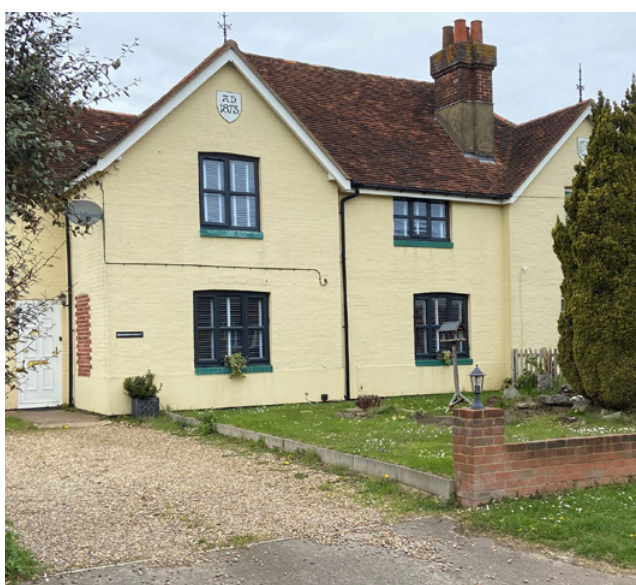
Period building with red clay tile roof and chimney stack being a key feature in the roofscape
