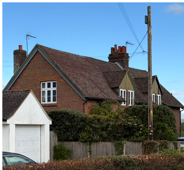
Simple pitched roof, in clay tiles, with dormers low on the roof line and punching through the eaves
