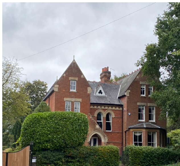
Victorian building with slate roof, which is in keeping with the architectural style
