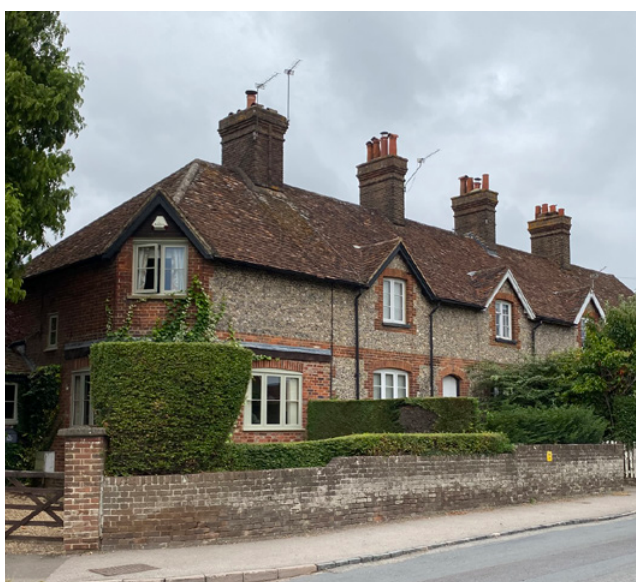
Period building with simple pitched roof and wall dormers and a lower eave line to the roof
