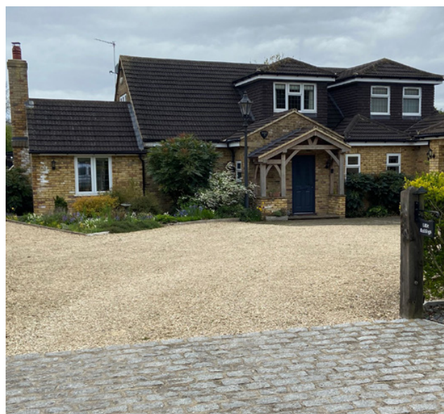
Single storey property in Whelpley hill, with later extension into the roof space
