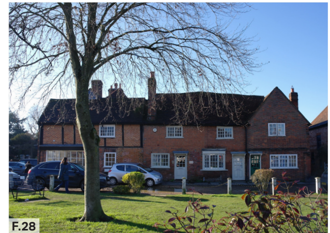
Figure 28: Aylesbury End, terrace houses grade II listed.
