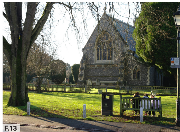
Figure 13: St Marys and All Saints Church, Grade II* listed.
