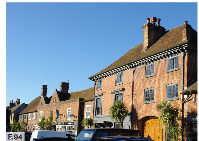
Figure 94: Varied roofscape within the historic core.
