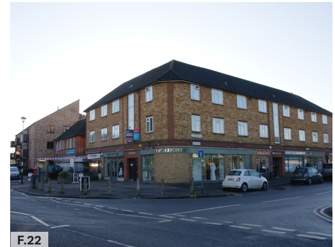
Figure 22: 3 storey building with retail ground floor and flats above in Holtspur.
