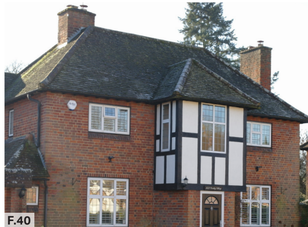
Figure 40: Chimneys at either end of the building using the same material as the main building.
