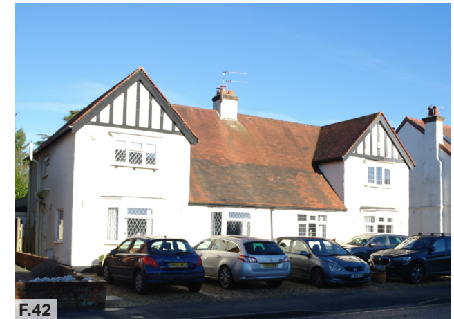
Figure 42: Chimney located centrally along the buildings roof.
