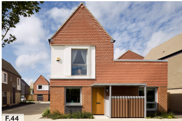
Figure 44: Example images showing bins are stored in the front of the house in a discrete way.
