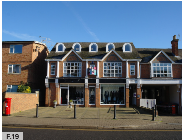
Figure 19: 2.3 storey building within the New Town.
