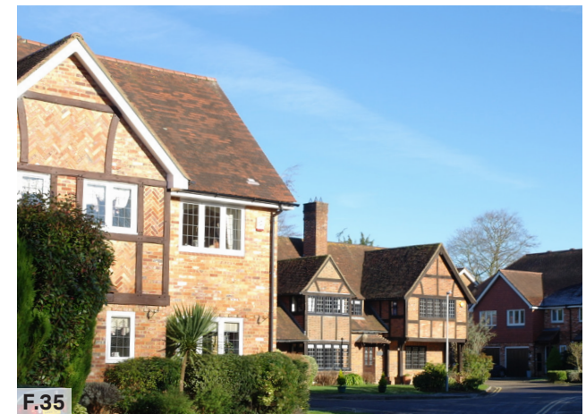
Figure 35: Multiple pitched roofs on residential buildings in the New Town.
