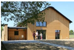
Wereham Village Hall, Norfolk Image Source: Passivhaus Trust
