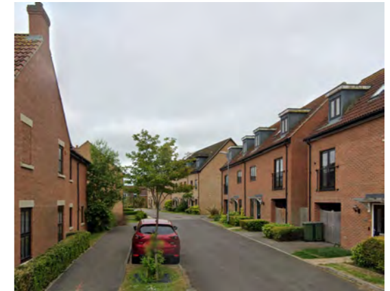
Parking here does not dominate the street scene. Limited on street parking with access to the rear of properties via gated undercroft areas.
