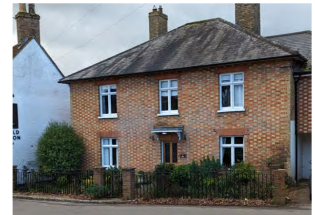
Metal railings with brick post soften by vegetation behind.
