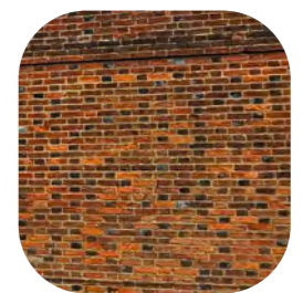
Red multi-brick, with burnt headers in Flemish Bond with first floor string course.
