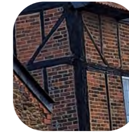
Timber framing, infilled with multi-red brick.
