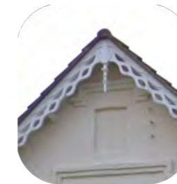
Decorative bargeboards finished with finials.
