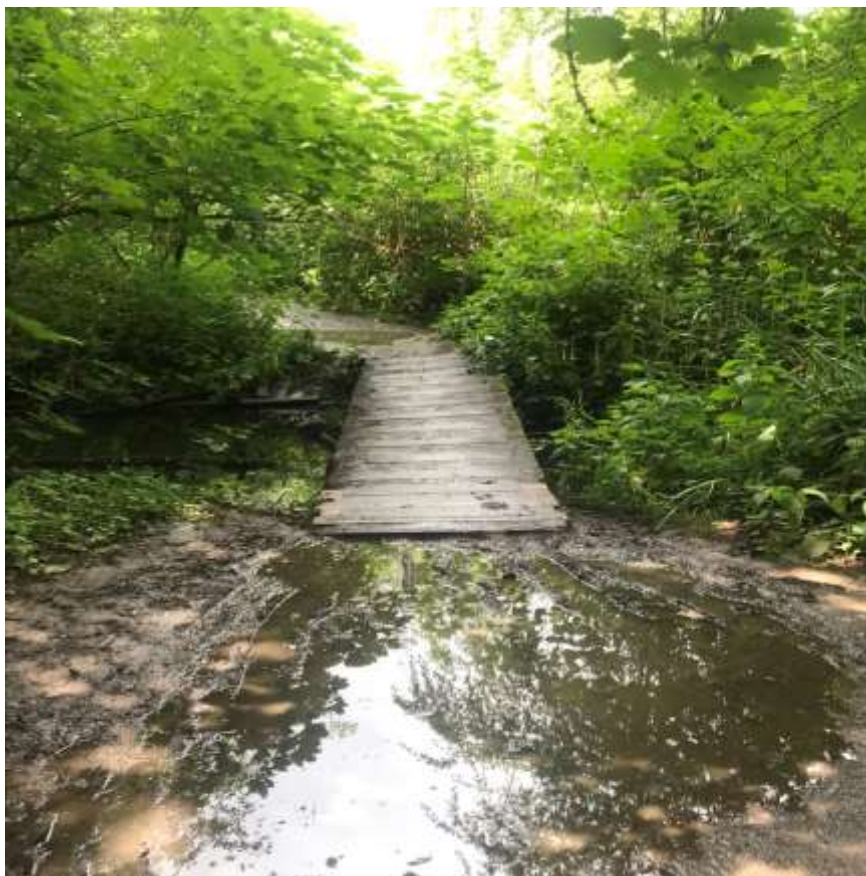
Figure 7: Footpath leading past the Crowne Plaza, connecting the Thames Path with the area around Westhorpe House (location 7 in table). This view northward shows parts of the muddy track, an old slippery footbridge and overgrowth.
