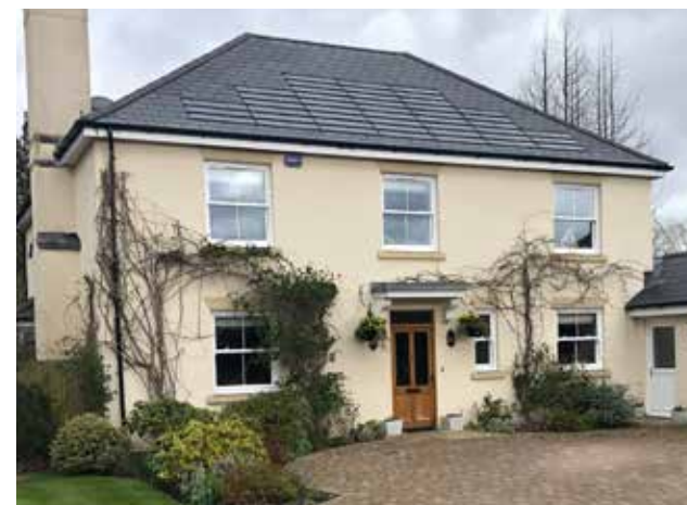
Figure 58: Use of shingle-like solar panels on a slate roof, with the design and colour of the solar panels matching those of the adjacent slate tiles (elsewhere in the UK).
