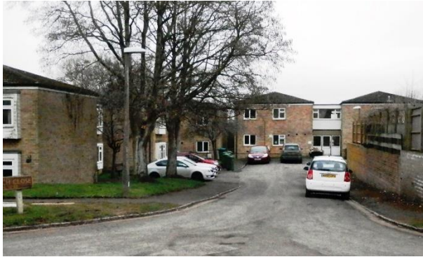
Church Close – Flats, close with extensive parking at rear, trees retained, grass verges
