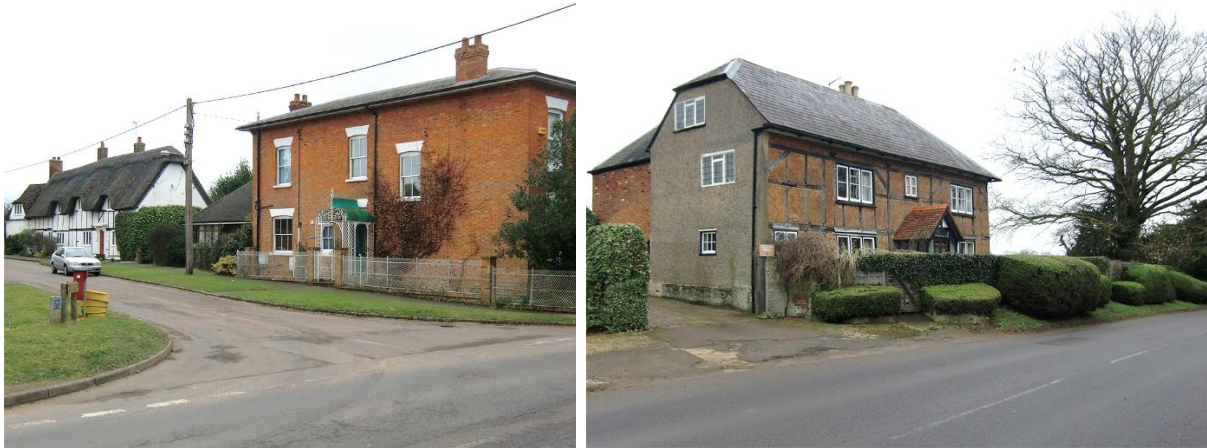
Chase House and Old Timbers, Cooks Lane, and Cedars Farmhouse (PW)
