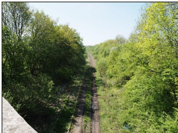
Salden Cutting before work to reopen the East-West Railway line – a perfect linear nature reserve
