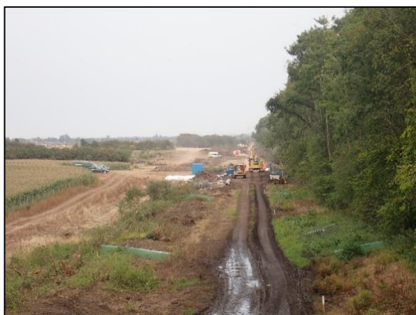
Work underway on the East-West Railway line adjacent to Salden Wood
