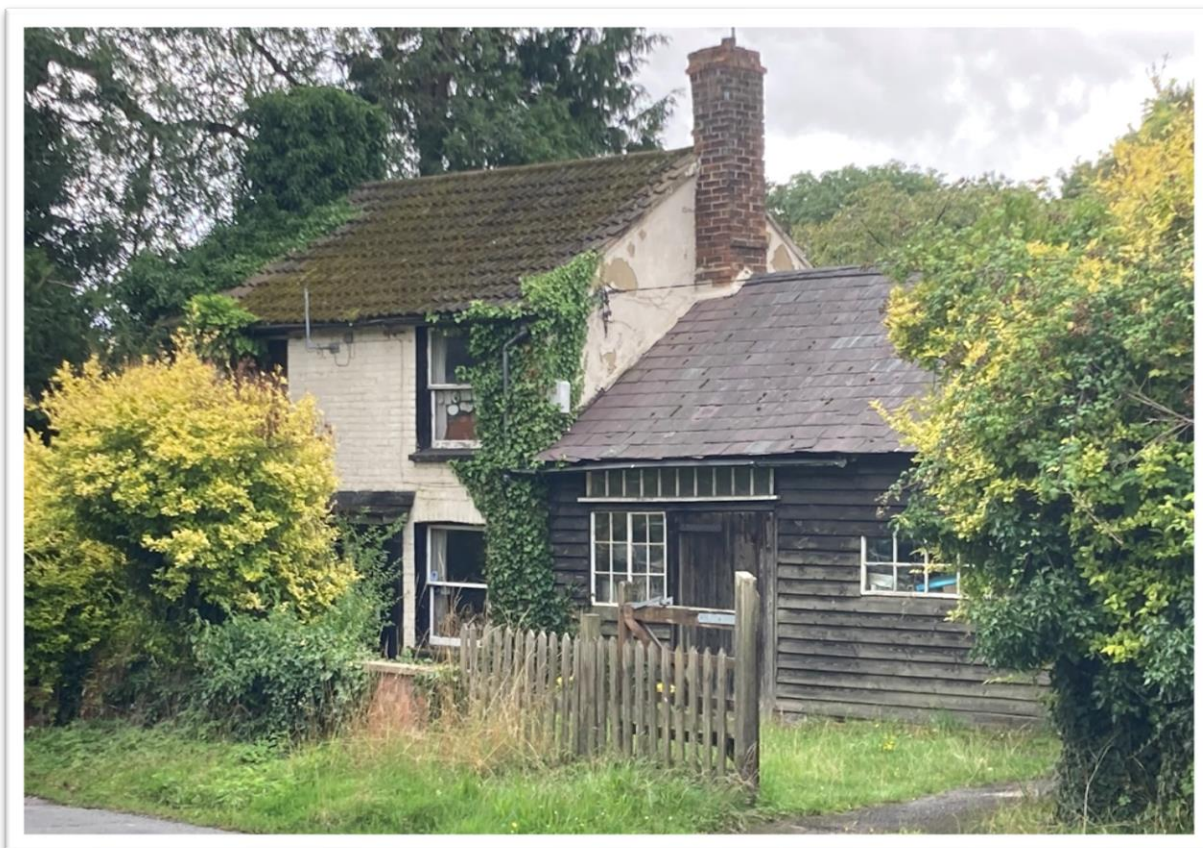
2 Stoke Road on the corner of Drayton Road, within the Conservation Area
