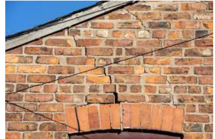
Subsidence cracks – sign of a problem
