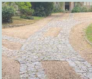
Mix of gravel and paving
