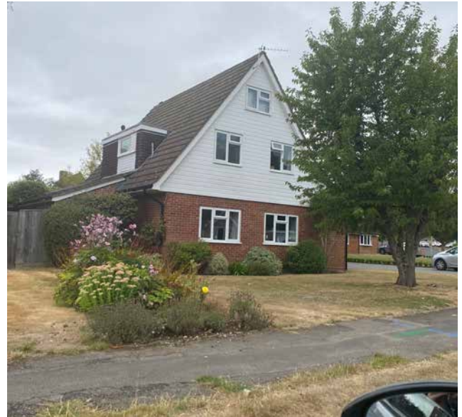
Figure 48: House on the Mynchen estate with distinctive pitched roof
