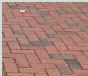
Herringbone brick paving
