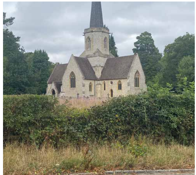
Figure 61: The Holy Trinity Church, located within the Penn Street Conservation Area.
