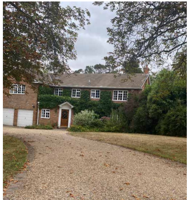
Figure 60: Example of a detached house in Knotty Green.
