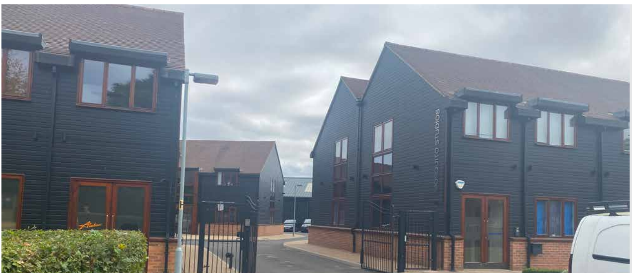
Figure 90: Black weatherboarding is used on Penn Street business park to try to create a barn aesthetic.
