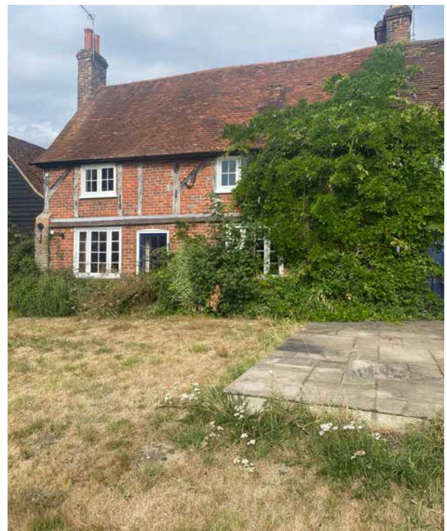
Figure 26: Listed building 'Fagnall Farmhouse'
