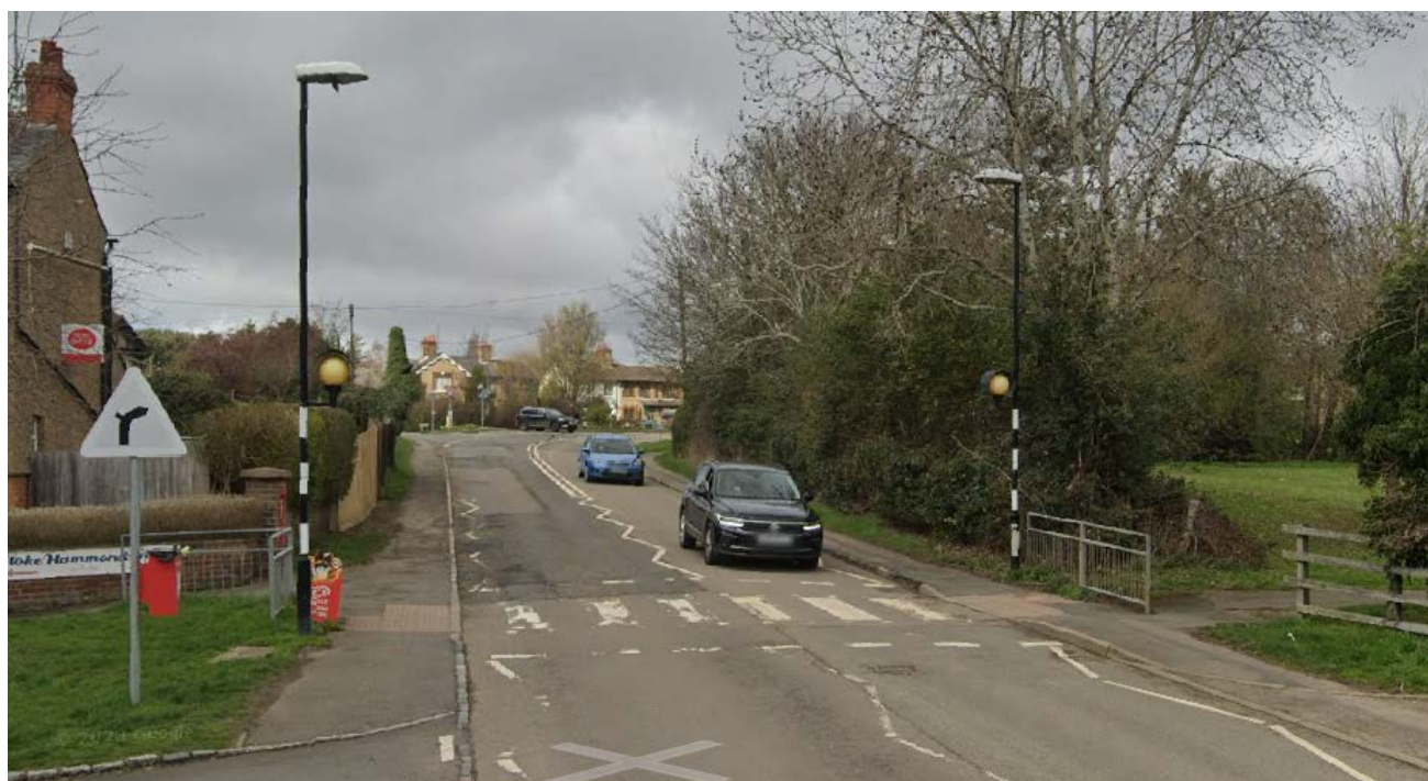
PEDESTRIAN CROSSING APPROACH FROM THE SOUTH
