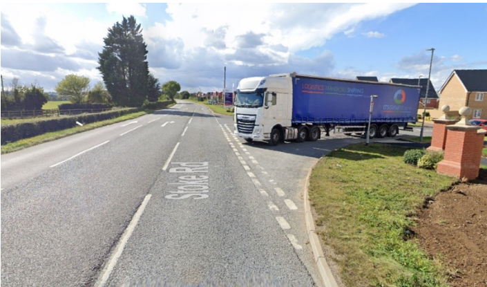
NEWTON LEYS SOUTH ENTRANCE LOOKING WEST
