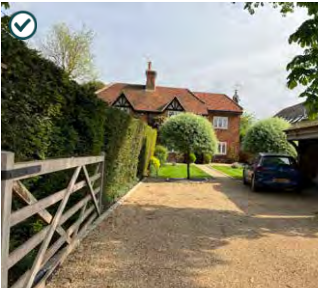
Figure 41: Positive example of boundary treatment using hedges and timber gate.
