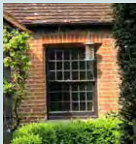
Dark walnut timber sash window
