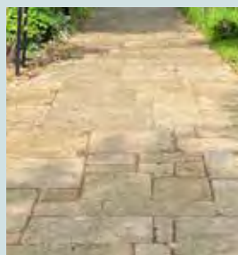
Permeable block paving
