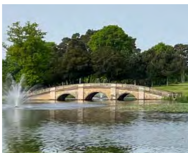
Figure 08: Stoke Park Bridge (Repton Bridge), Grade II* listed.
