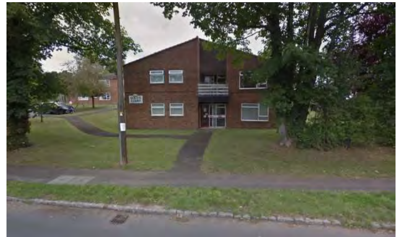
Site frontage to Rogers Lane
