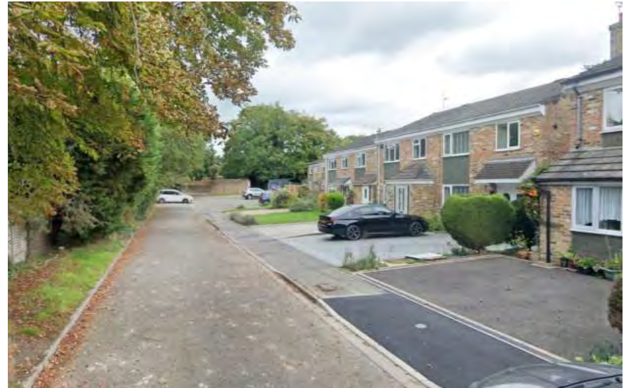
Existing building typology along Neville Close
