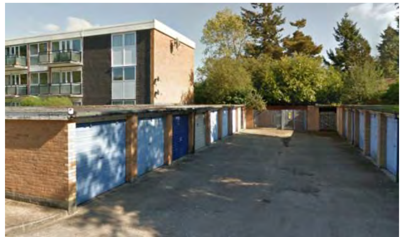
Garage site with sub station access
