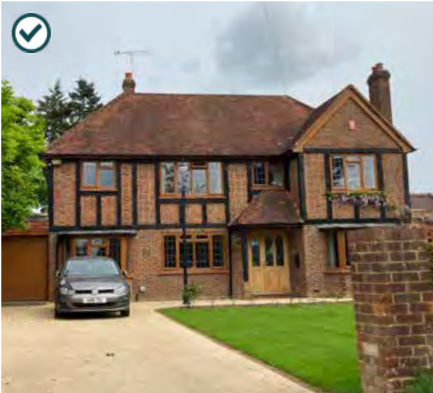
Figure 39: Positive example of use of materials and fenestration details which add to the character of the parish.
