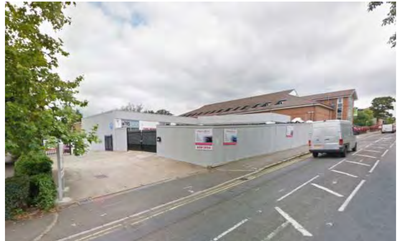
Site frontage to Bells Hill
