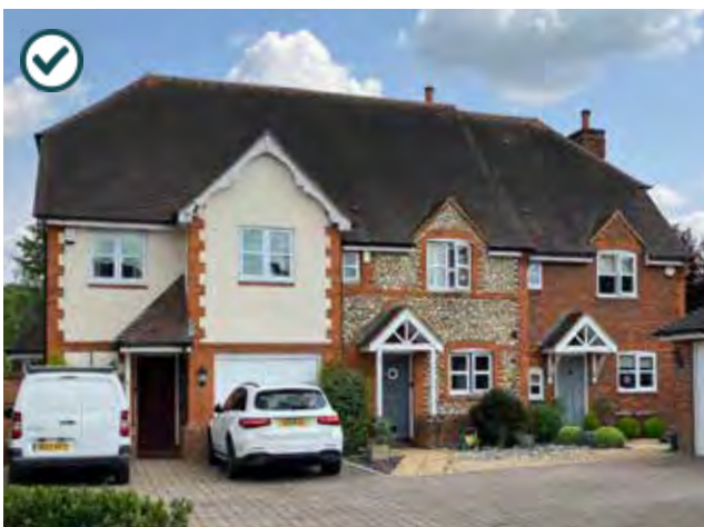
Figure 31: Positive example of use of fenestration and detailing within a new development. The mixed use of materiality (red brick, render, flint), variation in the building lines, quoins detailing, gabled front door canopy create a locally distinctive design.
