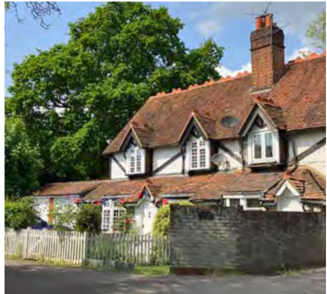
Figure 25: Cherrytree Cottage, Beaconsfield Road.
