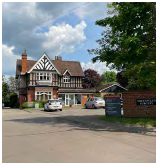
Figure 20: Southmead Surgery, Medical centre. Red brick on ground floor, and upper floor rough-cast and timber framework.
