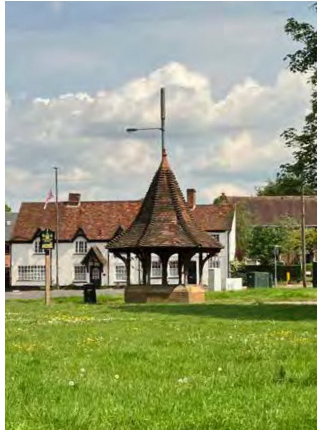
Figure 06: The Pump Shelter, Farnham Park
