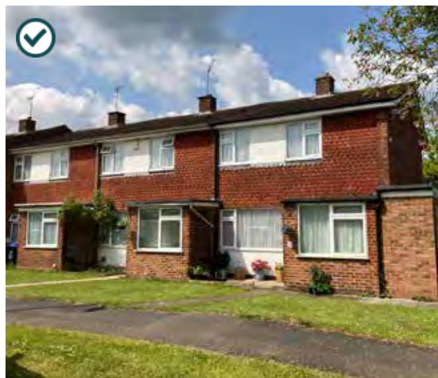
Figure 44: Housing mix could also be introduced through more recent interpretation of the terrace typology
