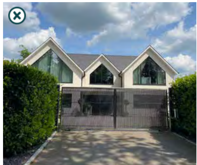
Figure 40: Negative example using unsympathetic material palette, out of proportion windows
