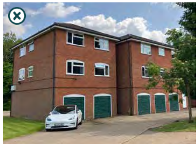
Figure 32: Generic building style within a new development. The lack of fenestration and detailing creates a non-specific feel.
