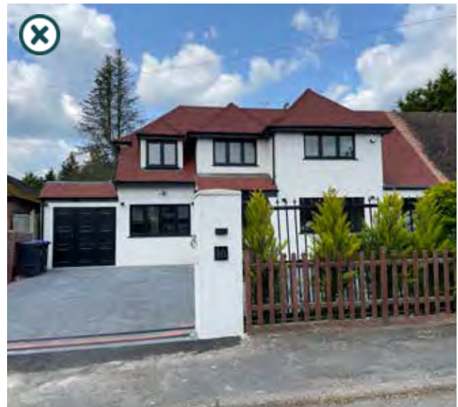
Figure 30: Negative example of hipped roofs. The set of hipped roofs placed uniformly in a row, adding an out-of-proportion feel to the roof and lacks interest in the roofscape.
