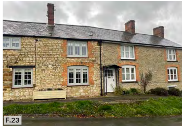
Figure 23: Row of Rubblestone cottages with red brick detail, Fulwell Road.
