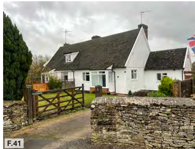
Figure 41: Example of dormer bungalow, corner of Fulwell Road and Orchard Place.
