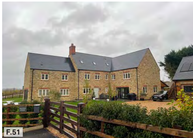
Figure 51: New development on the site of Mill Lane Farm in the traditional style of the village using rubblestone facades.
