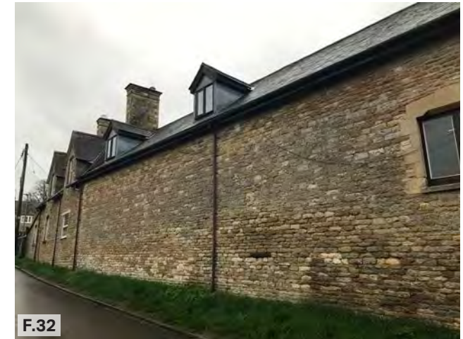
Figure 32: Example of rubblestone facade with dormer windows, Beachborough Prep School, Mill Lane.
