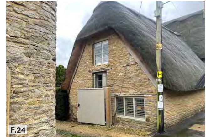
Figure 24: Gable end of grade II listed dwelling on Main Street.
