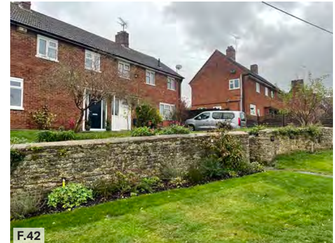
Figure 42: Two storey semi-detached dwellings on Orchard Place.
