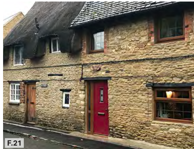
Figure 21: Terraced cottages, Main Street.
