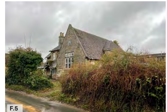
Figure 05: Derelict school building on Main Street.
