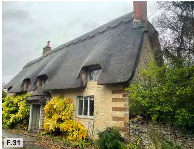
Figure 31: Little Thatches, Mill Lane.
