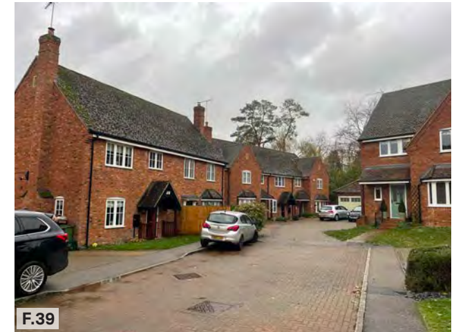
Figure 39: Internal view of semi-detached dwellings in School Close, Mill Lane.
