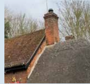
Chimney stack built by red brick
