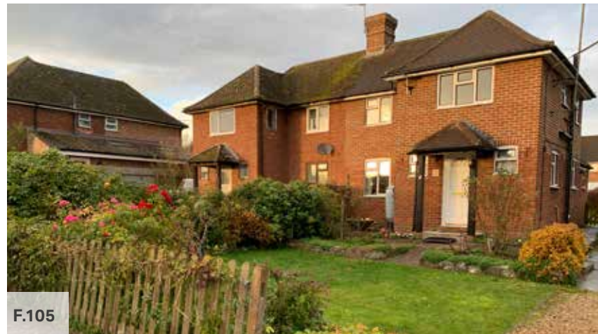
Figure 103: Priory Hotel a detached building on the High Street built by red brick and timber frame and multi pane casement windows
