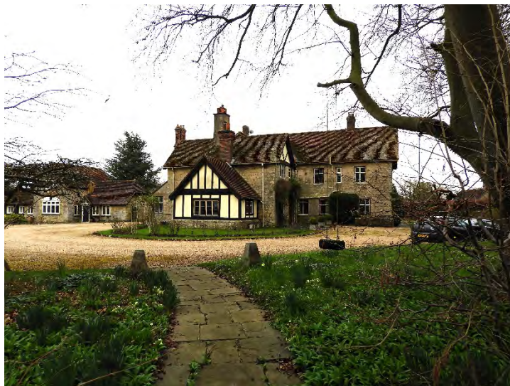
View of the rear of the listed building and wide drive that separates it from the rear garden and proposed allocation plot.
