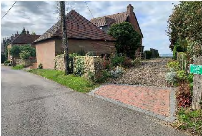
Fig. 3 existing vehicle access
