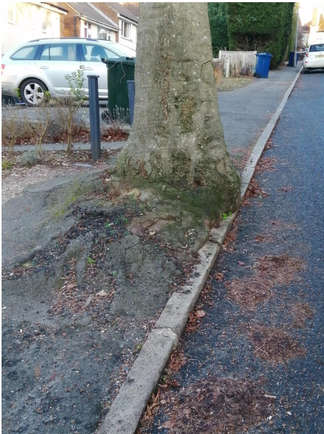
Figure 27: the kerbstones remain in place beside tree T016, but the narrowness and pronounced mounding of the pavement means there is no easy passage for pedestrians.
