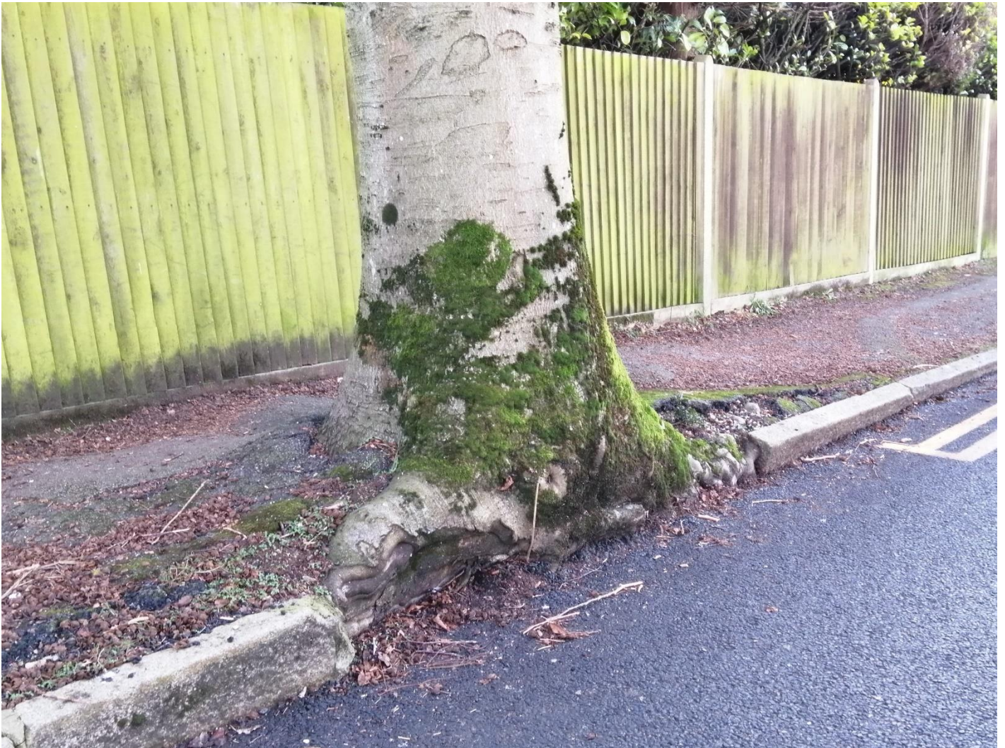
Figure 25: the beech tree T013, showing buttress roots occupying the space vacated by kerbstones. Space for pedestrians between the tree and the boundary fence is limited.
