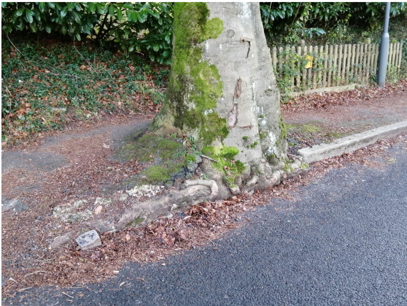
Figure 26: Tree T015, showing limited space for pedestrian passage between the tree and the property boundary behind. Buttress roots have filled the space where kerbstones may once have been.
