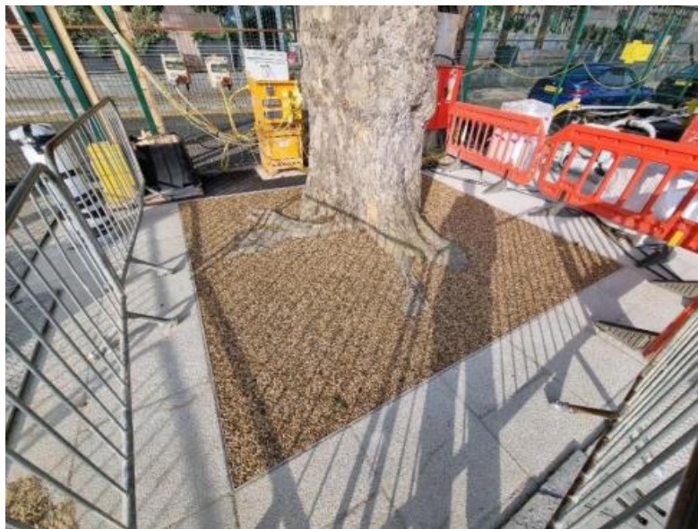
Figure 2 - Flexi-Pave Tree Pit installation
